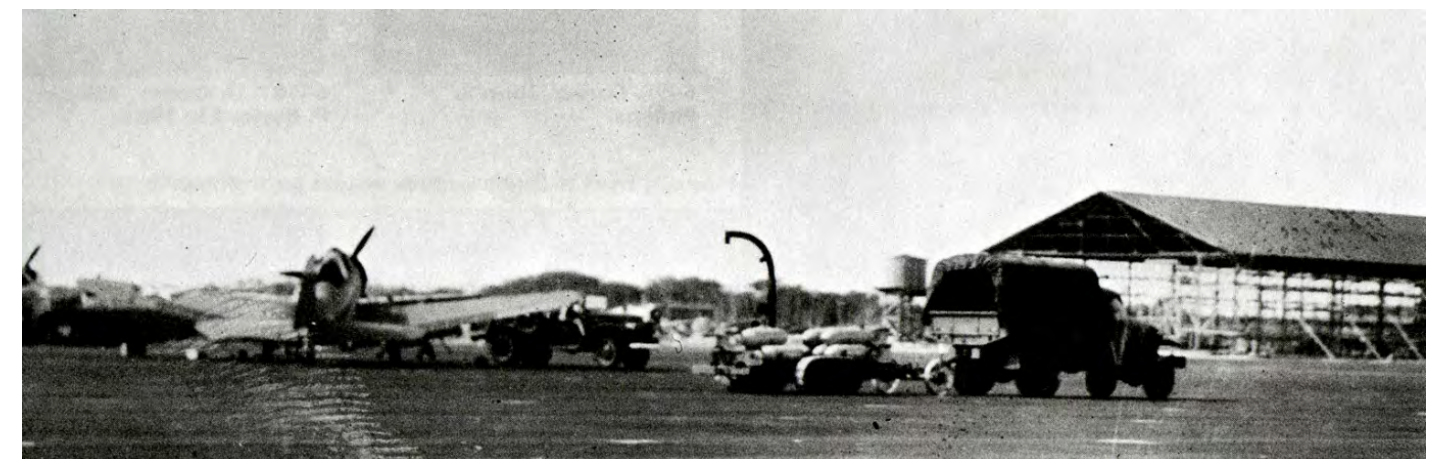
Hangar under construction (Credit: Goldstein and Dillon, 1991)
