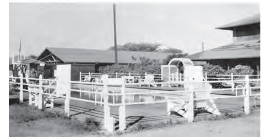
Finished swimming pool adjacent to recreation building
