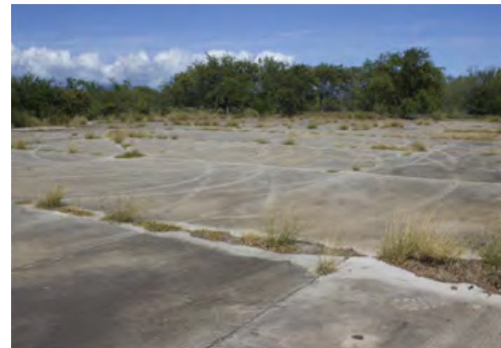
Concrete Warming-Up Mat (present day). (Credit: AECOM)
