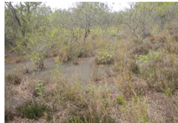
Runways are deteriorating from vegetative growth, weather, other factors.
