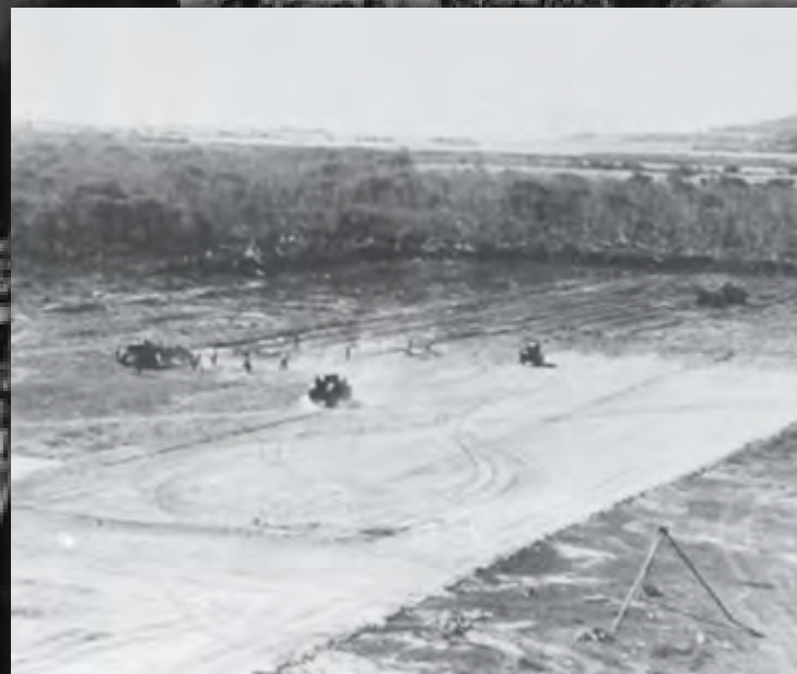
Preparing the runway 1940
