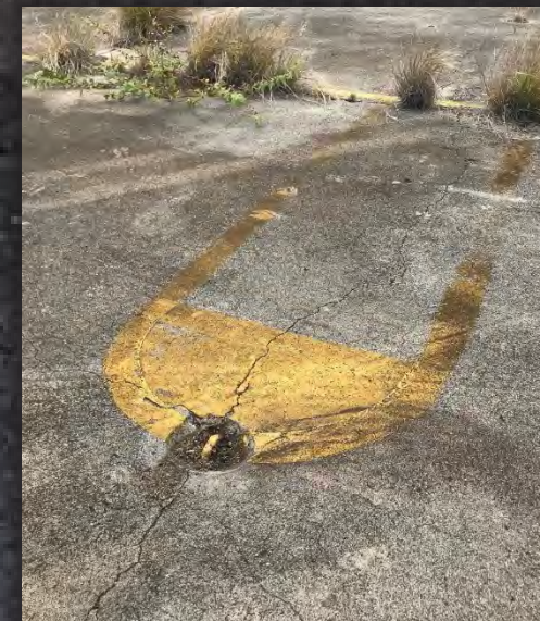
Metal tie down on mooring apron.
