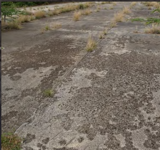
Damage to concrete Warm-up Platform from Japanese strafing.
